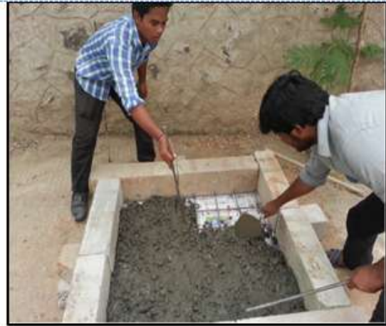
Fig.3 Placing of Concrete
