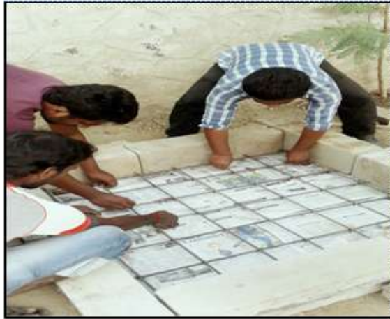
Fig.2 Fixing of Reinforcements
