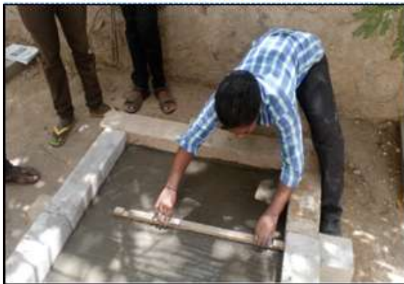
Fig.4 Finishing of Concrete
